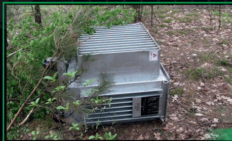
The damage made by thieves at stealing components of the transformer (oil cooling, non-ferrous metals).
