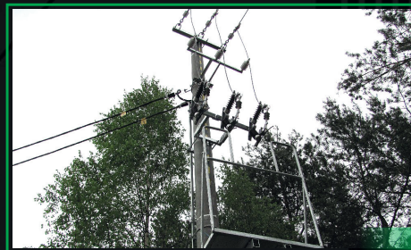
The damage made by thieves at stealing components of the transformer (oil cooling, non-ferrous metals).
